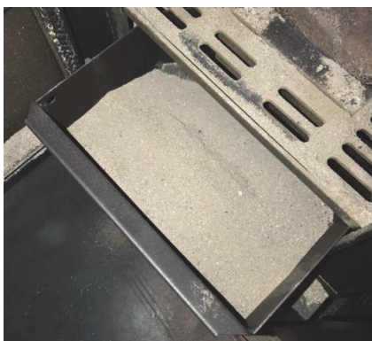
Example of dirty ash box
