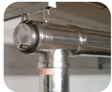
Tee Cap with drain used to provide condensate drain location.
