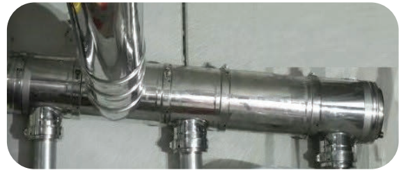
Tee Cap with drain used to provide condensate drain location.
